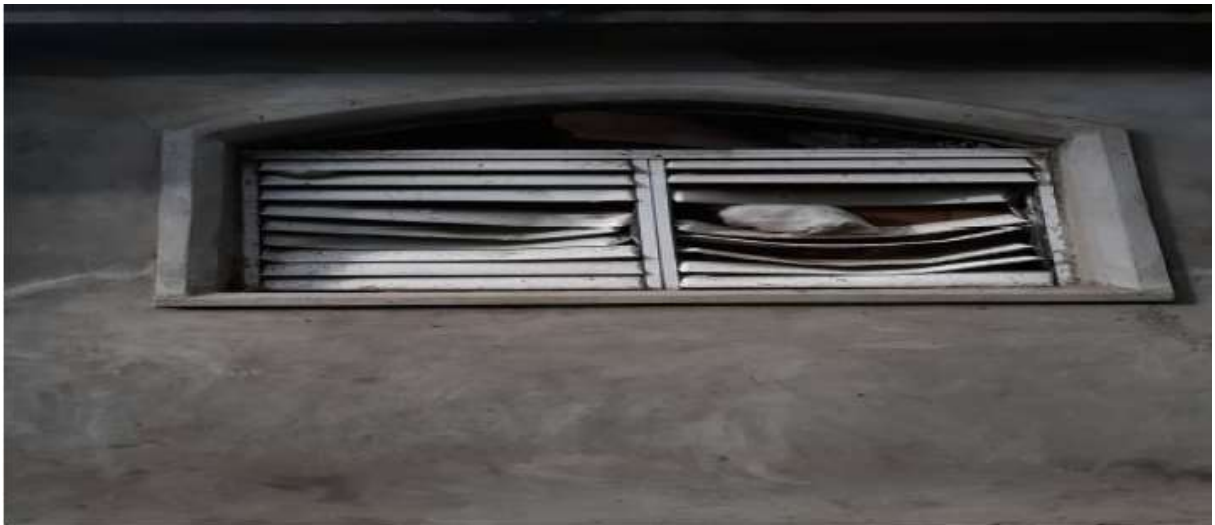
Figure 5: A picture of one of the windows broken during the attack.
